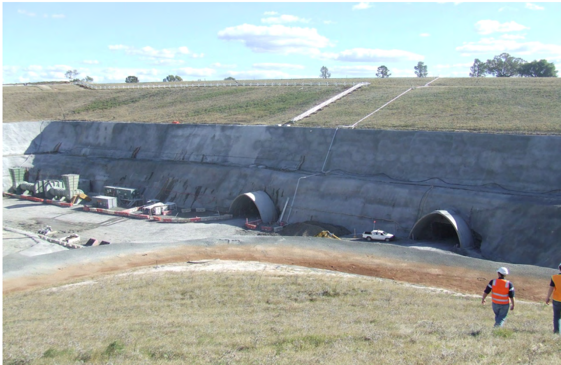
Plate 6: Three Portals within Box Cut – Narrabri Underground Coal Mine – April 2009
